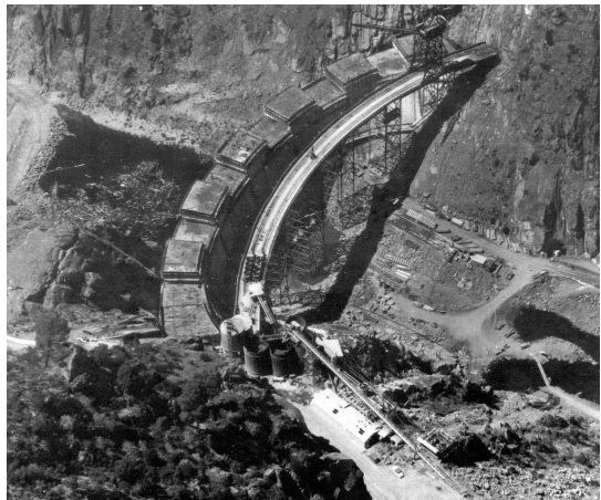
Construction of Monticello Dam.
