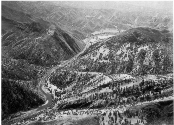
Devil's Gate before the construction of Monticello Dam. Cold Canyon is near center on the left edge, and Berryessa Valley and Putah Creek can be seen beyond the "gate."
