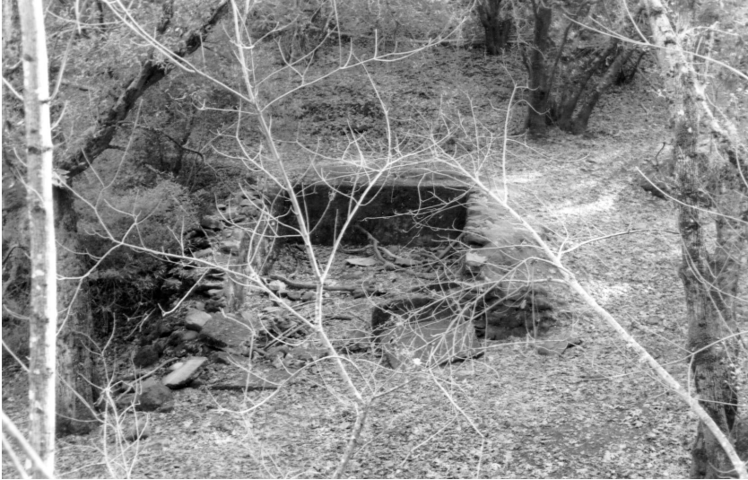
The remains of the Vlahos' cold storage.
