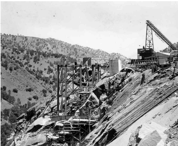
Monticello Dam Construction, 1956
