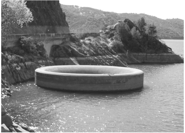
The spillway at a low lake level.
