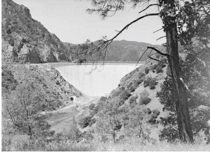
Monticello Dam looking west. Pre-hydroelectric power plant, 1958. The spillway is clearly visible on the bottom left of the dam.
